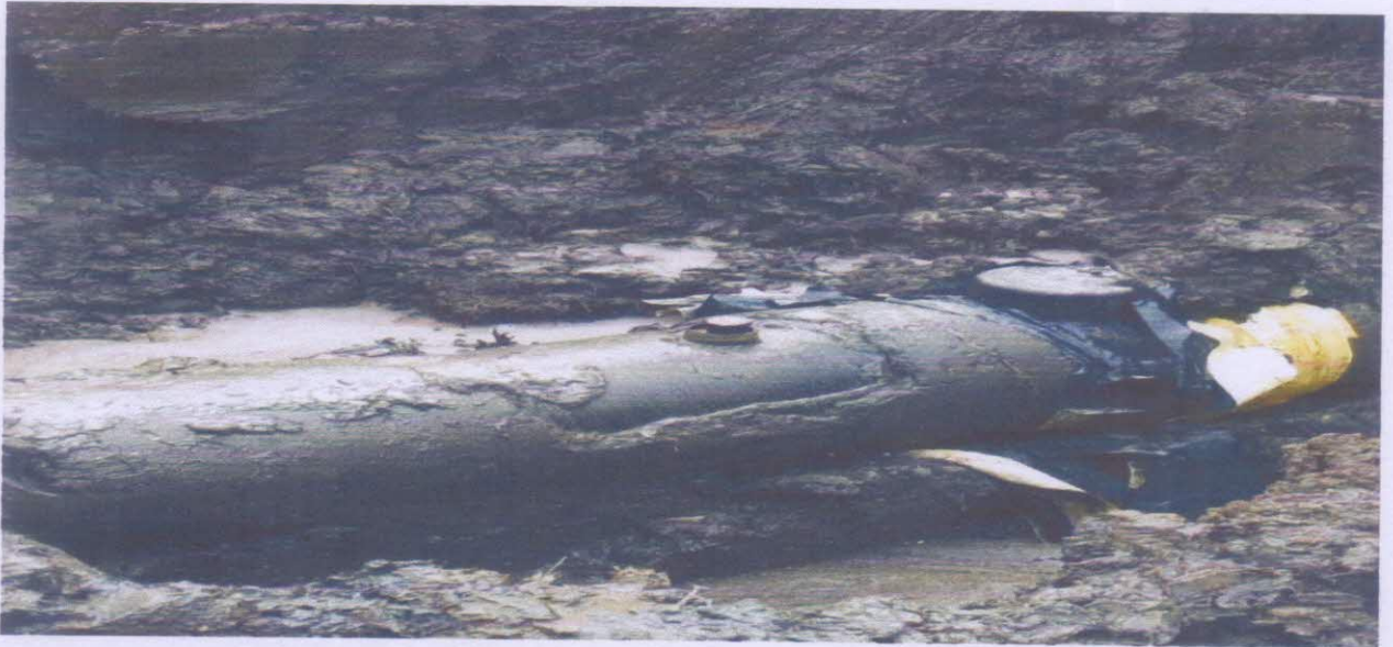
SPILL POINT AFTER EXCAVATION SHOWN
